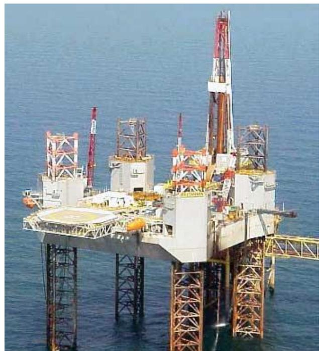
installed at the WSH location. It is well suited to the harsh operating conditions of the Bass Strait and, once converted to a MOPU with production facilities, its size will allow deck space for drilling of the WSH production and exploration wells with the use of a de-mountable modular platform rig.
